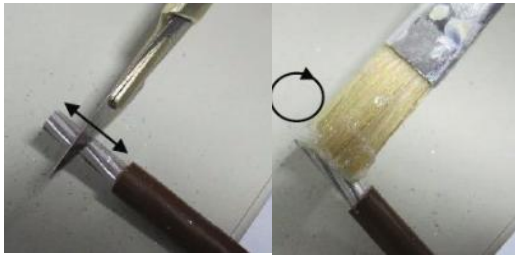
Figure 3-38 Preparing Aluminum Conductors prior to connecting
