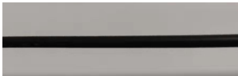
Fig. 7: view of cables
