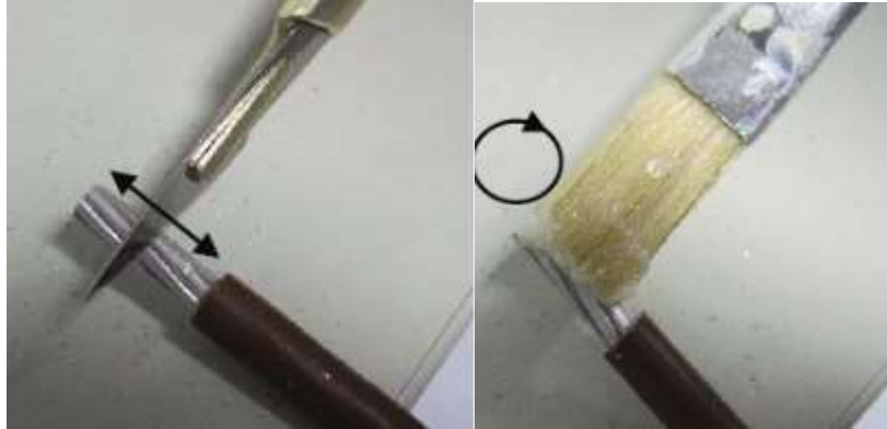
Figure 3-30 Preparing Aluminum Conductors prior to connecting
