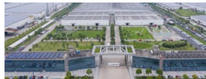
Haining Solar Intelligent Factory China
