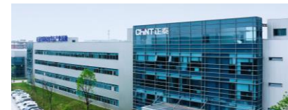
Power T&D Jiaxing Factory China
