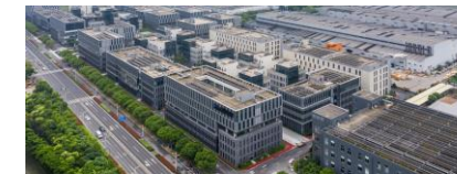
Power T&D Shanghai Factory China
